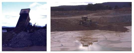
Figure 33: Capping tailings: (left) causing bow wave failure due to use of large mine-scale equipment; (right) loss of an excavator on too thin a cover over soft tailings
