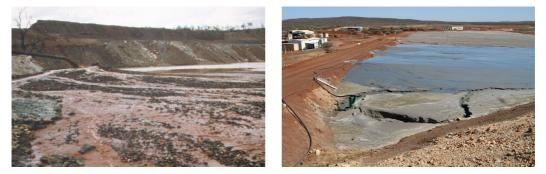
Figure 32: Capping tailings gradually using small-scale equipment: (left) surcharging tailings using small trucks; (right) pushing surcharge in thin lifts using a D6 Swamp Dozer
