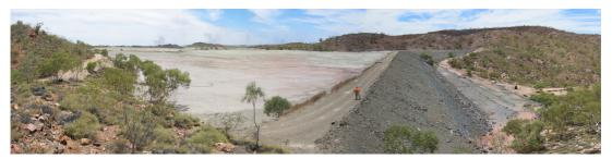
Figure 23: Tailings storage facility embankment in a wet climatic setting
