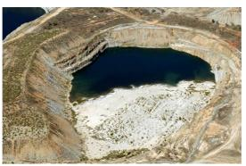
Figure 7: Co-disposed waste rock and thickened tailings in a completed open pit
