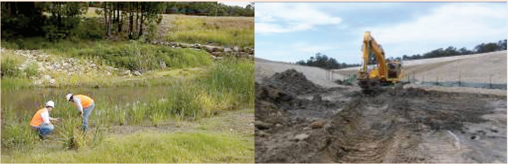
Preparations for Maryland Creek re-establishment.
