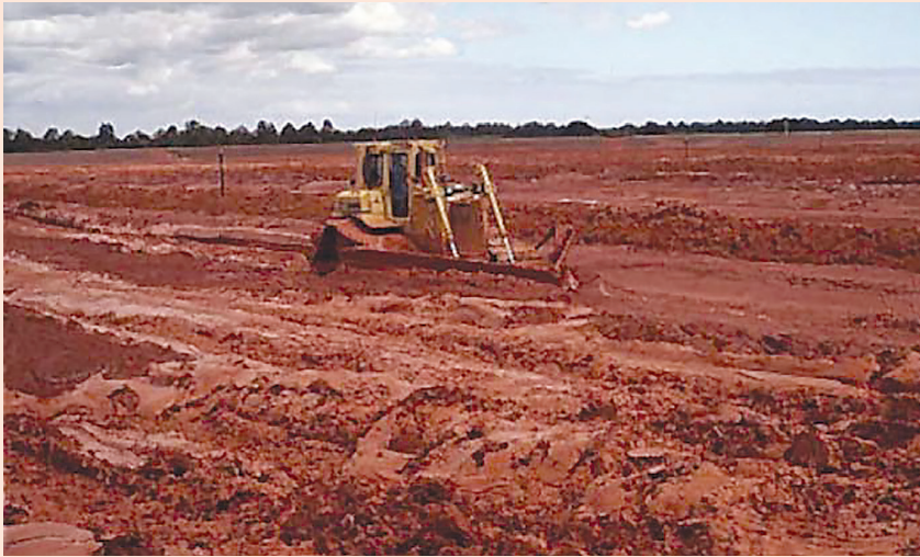
Using a D6 swamp dozer to enhance the drying rate.
