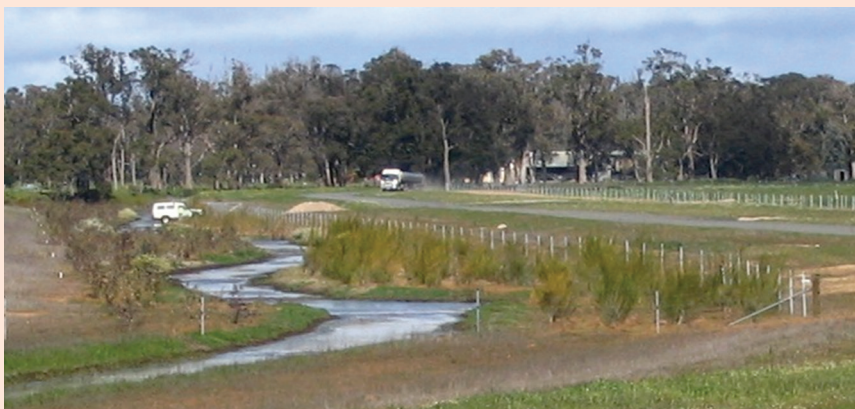
Reconstructed creek stabilised, showing stream rehabilitation circa 2008.
