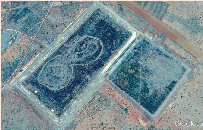
Three Cell TSF 2013—after 2008–09 rehabilitation. (Google Earth)
