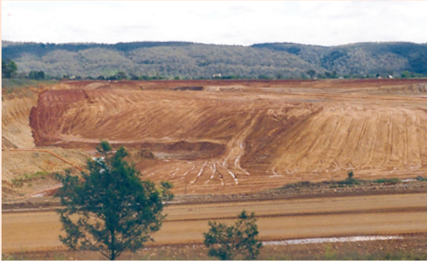
Penrith gravel pit rehabilitation in progress (October 1990).
