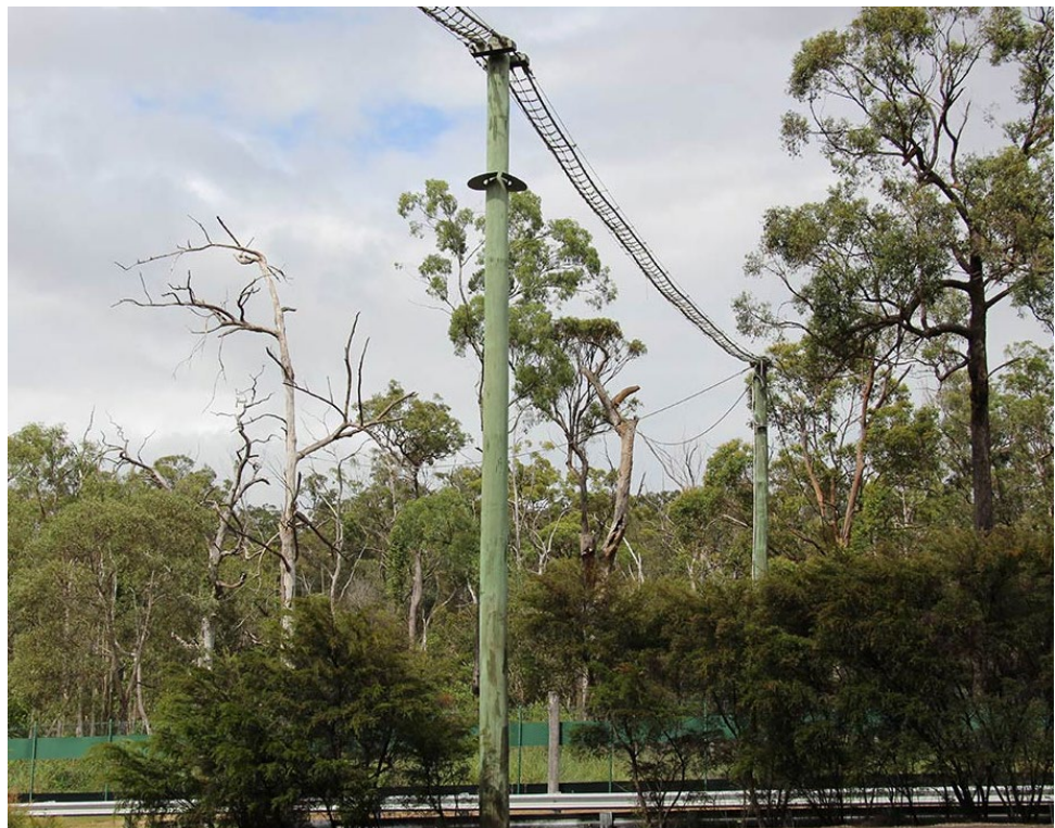
Plate 9. Overhead fauna crossing structures (source: Griffith University)
