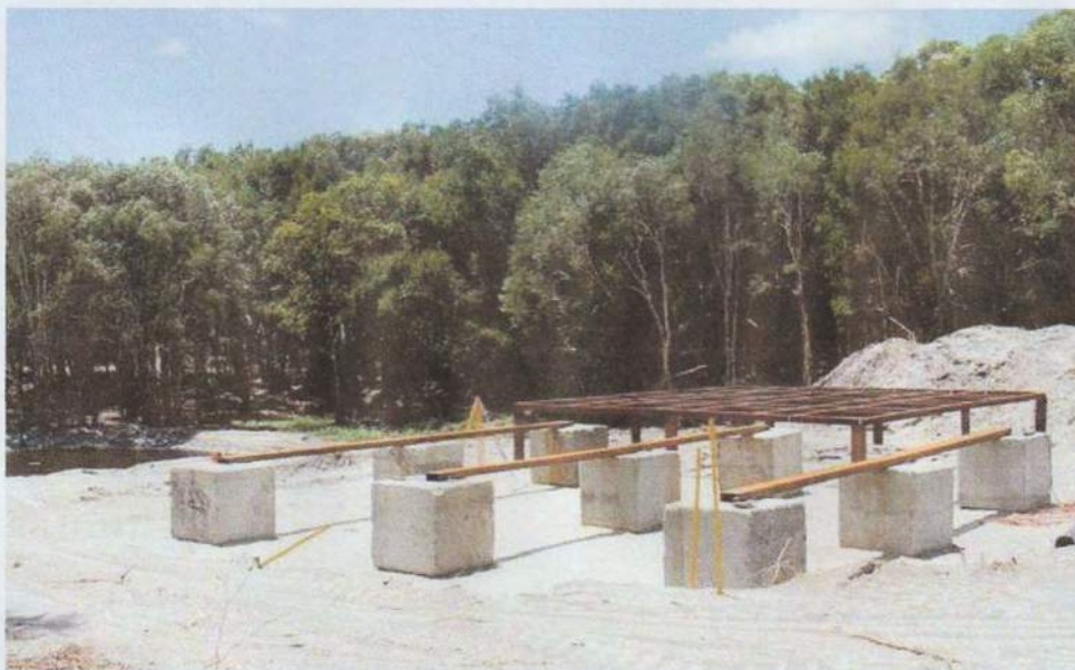
Beach conservation advocate Reg Lawler says a radiation clean-up seems to be underway at Inskip Point. Picture: Submitted
