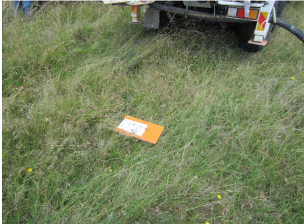
Photo 2: GS504 Before Drilling
