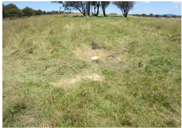
Photo 3: GS504 After Drilling
