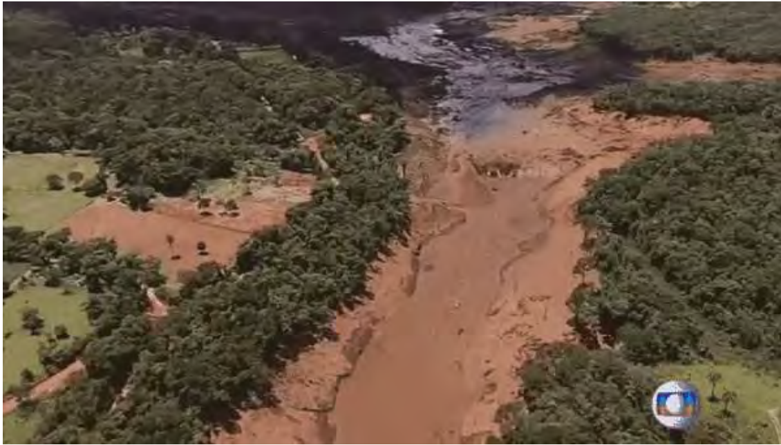
Figure 25: Vale Company TSF failure 2019
