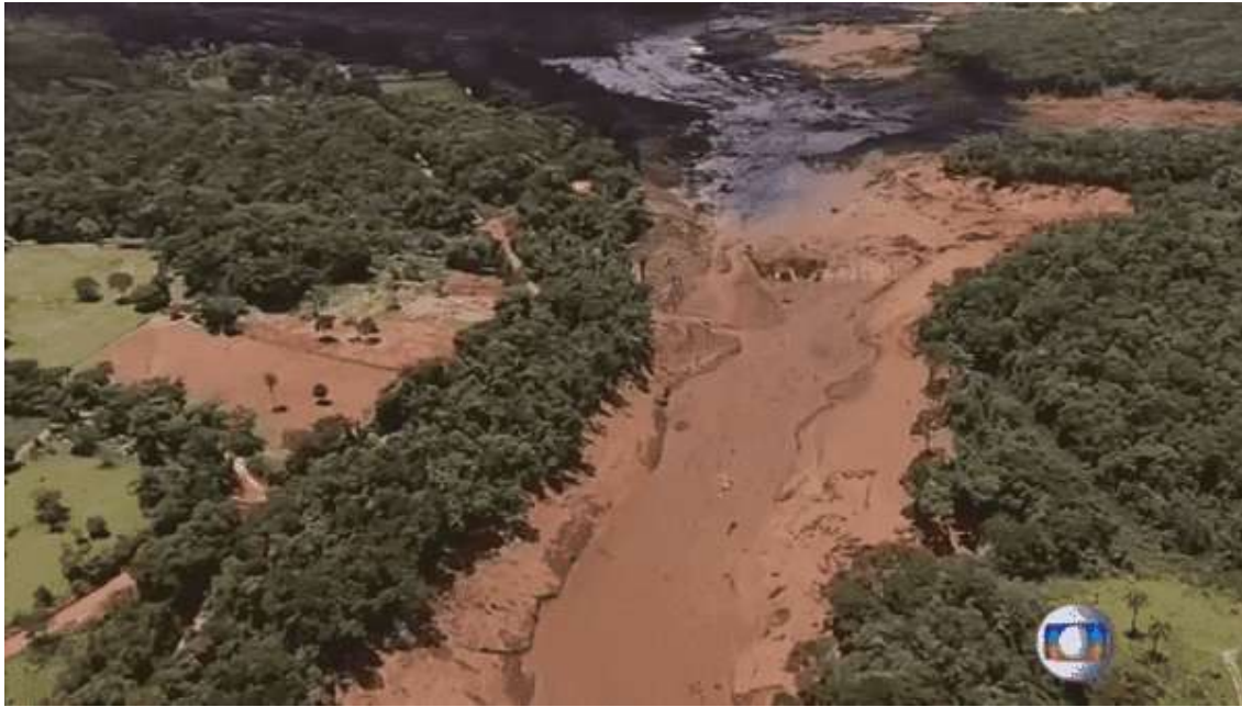
Figure 25: Vale Company TSF failure 2019
