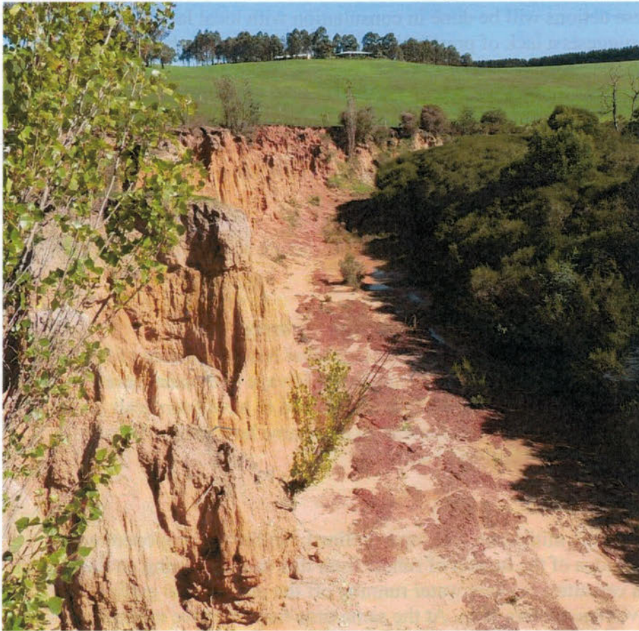
Photo 1 Erosion of Dispersive soils Moulin Creek
