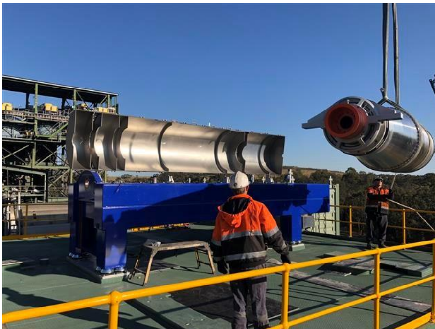
Rixs Creek, NSW – Coal Tailings installation
