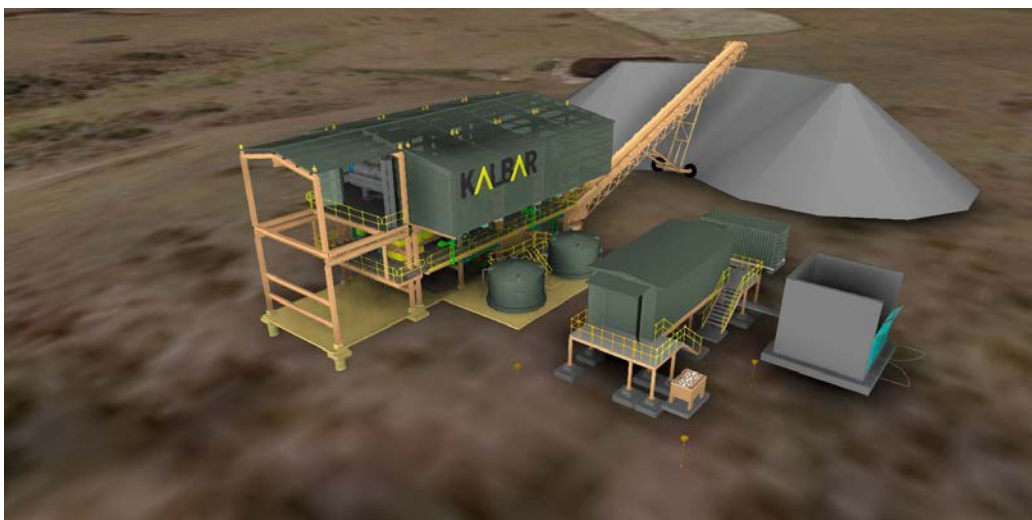
Figure 7 Centrifuge building and cake stockpile
