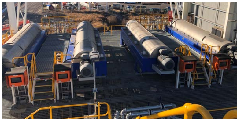
Figure 8: P3 Decanter (solid bowl) Centrifuges installed on a slimes dewatering duty
