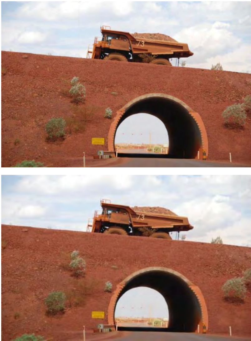
Figure 6-2: Corrugated-plate arch bridge structure
