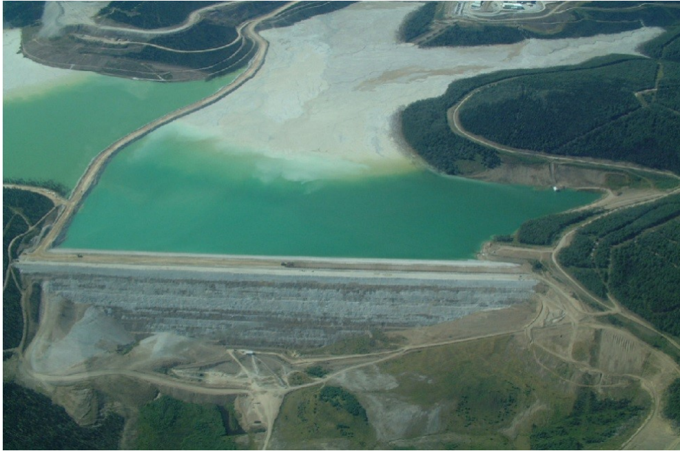
Figure 1 Wet tailings dam at Fort Knox mine near Fairbanks (Patagonia Under Siege 2018)
