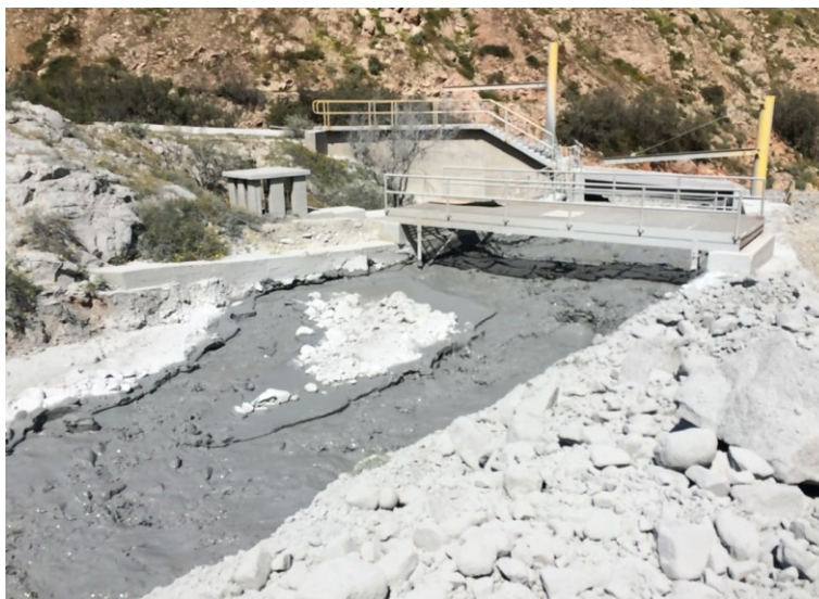
Figure 17 Existing tailings stream at Cuajone mine
