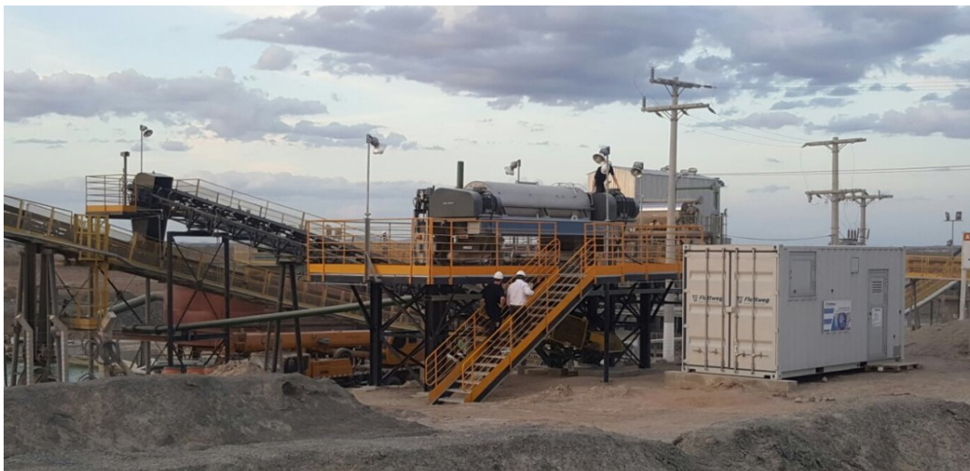
Figure 12 Centrifuge installation at Braúna mine
