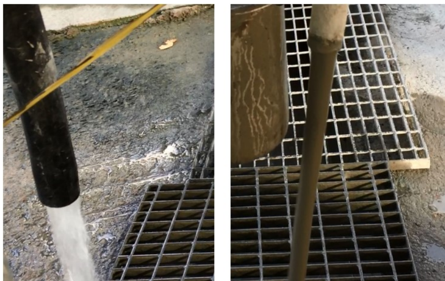
Figure 13 Centrate discharge and feed material
