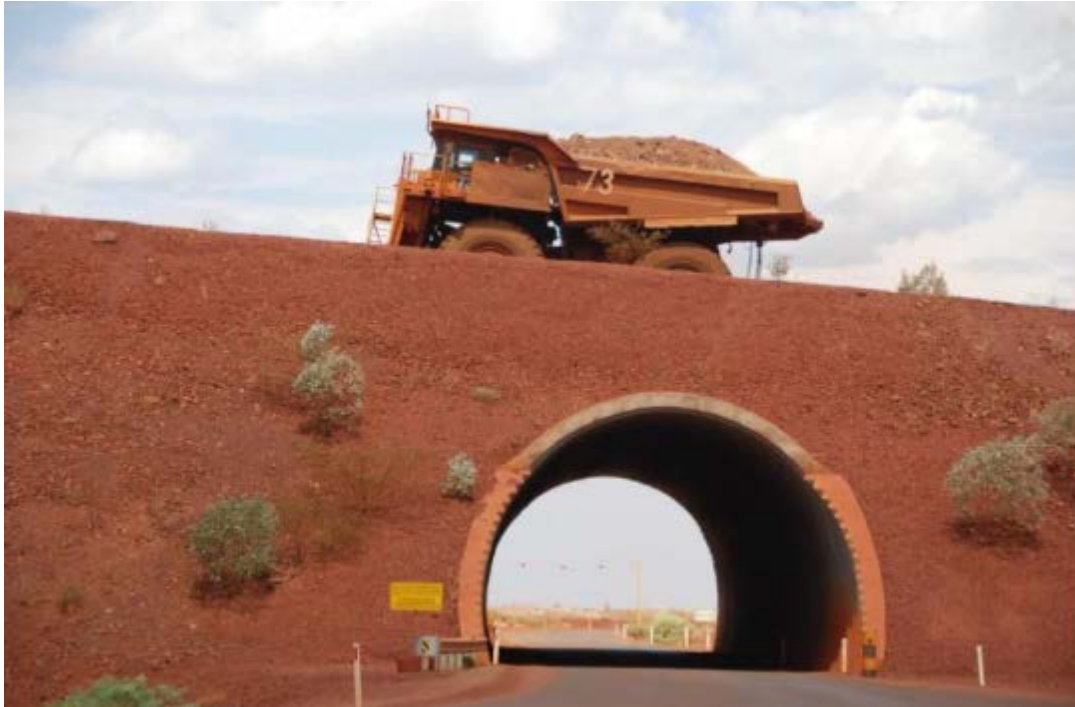
Figure 6-2: Corrugated-plate arch bridge structure
