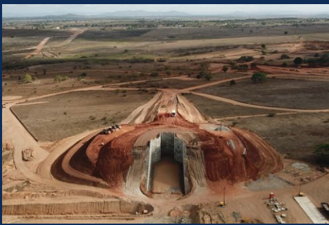
Primary crusher pad construction
