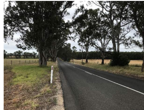
Site Access – View South
