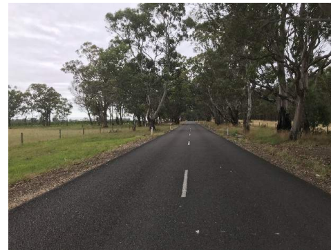
Haul Road Intersection – View South
