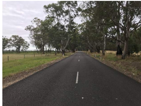
Haul Road Intersection – View South
