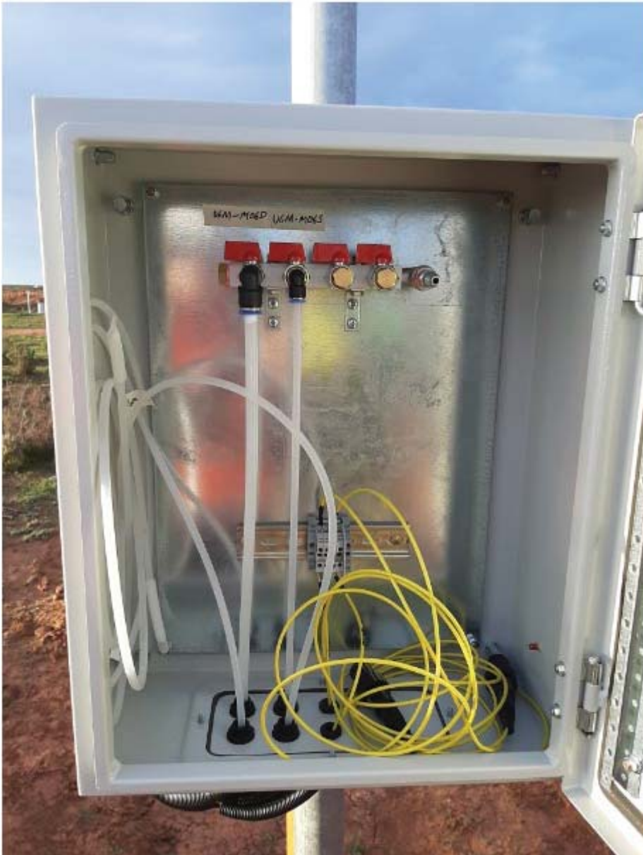
Plate 4.2 Specialised groundwater collection system – Sample collection setup
