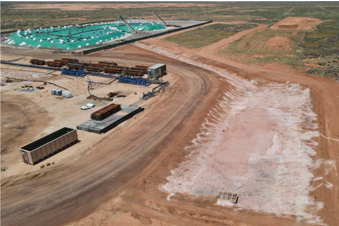
Photograph 10.5 Activity site pre-demobilisation – looking south (20 November 2020)
