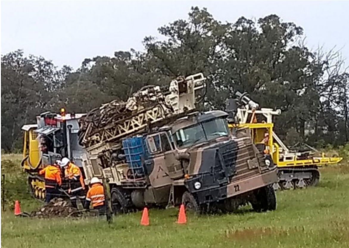
Bogged drill rig
