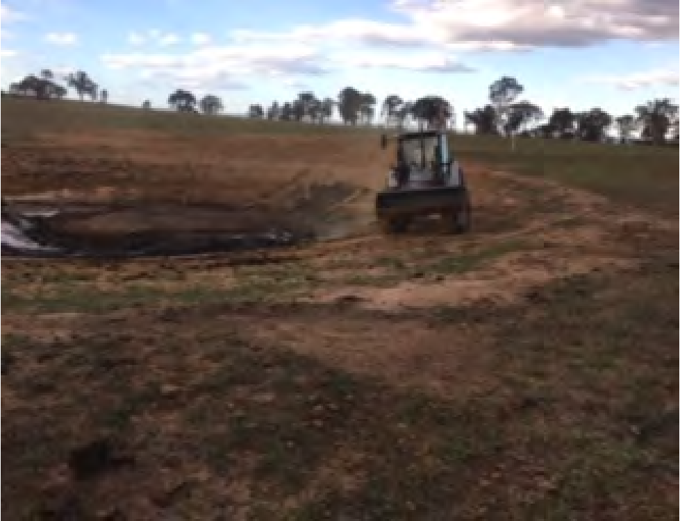
Cleaning out sediment accumulated in dam
